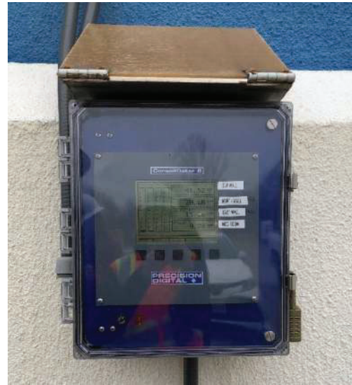
Figure 2-2 NCWWTP Bar Screen H 2 S Local Monitor
